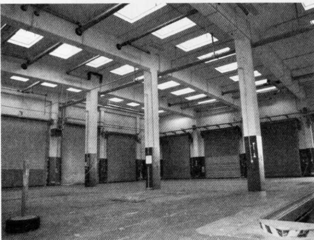
Huge vehicle repair bays in the vehicle maintenance building.
